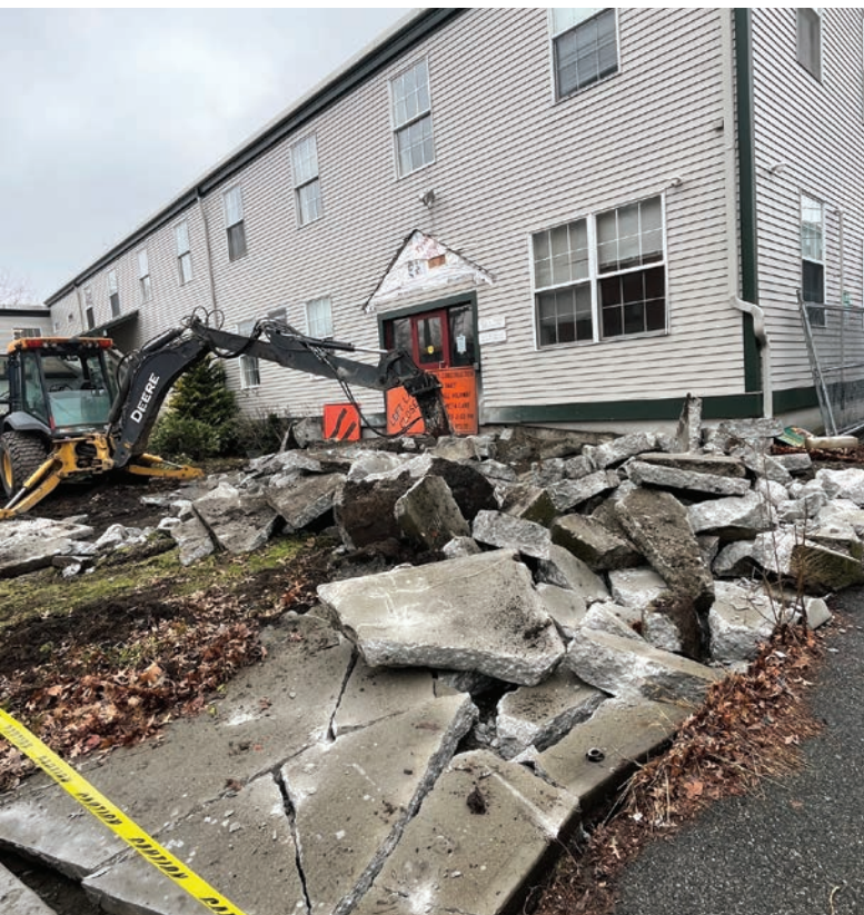
View of the building facade as the front steps and ramps were demolished.
