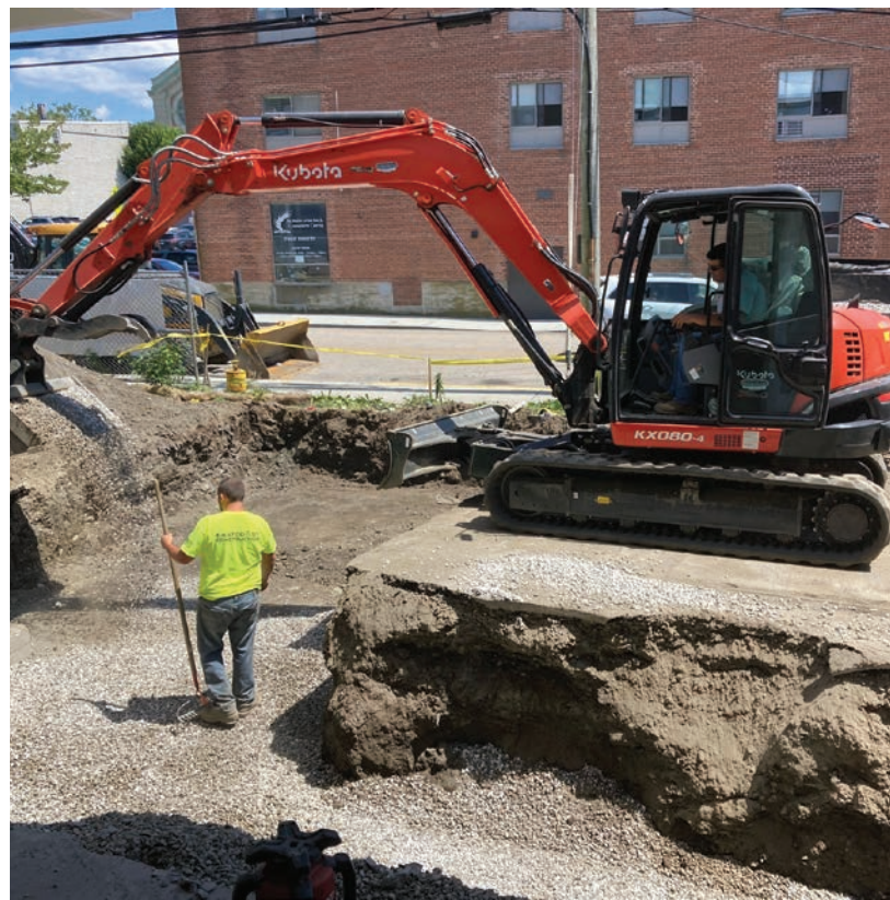
View from inside the old Receiving space as the loading dock is removed and the site regraded..
